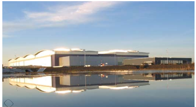
Figure 1. Assembly plant of Airbus A380 (Photograph E. Grimault)
