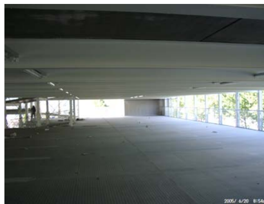
Figures 1 and 2. Outside and inside views of the car park
