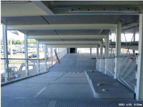
Figure 3: internal view with structure and ramp
